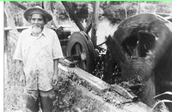
A traditional 5 kW Micro Hydro installation in the Tundagan village, Central Java, built by a local farmer (Bachri 2000).
