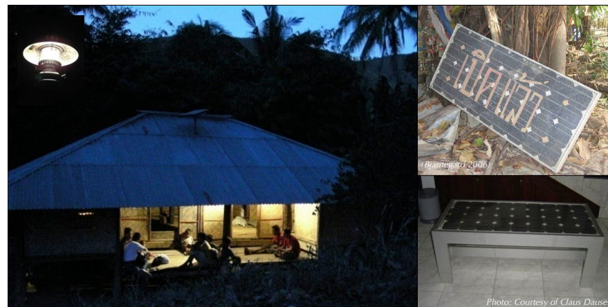
Malfunctioned PV system in Eastern Indonesia and Thailand
