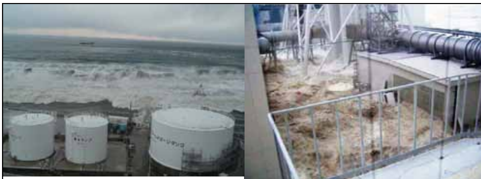
Tsunami impact on Fukushima Daiichi power station (Fukushima Daiichi Accident – Technical Causal Factor analysis, EPRI, March 2012)
