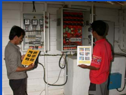
Induction Generator Controller PLTMH Cipaleubuh, Jawa Barat IGC HeksaHydro – 15 kW
