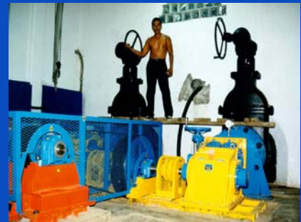
Bili-Bili, Gowa, Sulsel X-flow T-14, ELC-2x100 kW 1999
